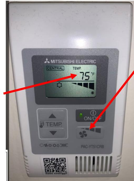
You can adjust the fan speed as well if desired, but the highest fan speed seems to work well for most spaces.
