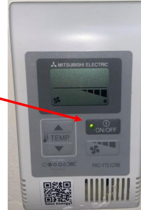
After a few minutes, the defaulted cooling set point of 85 will show on the screen. You must now press the down arrow to move the set point to your desired temperature. (remember, 75 is the campus low cooling set point).
