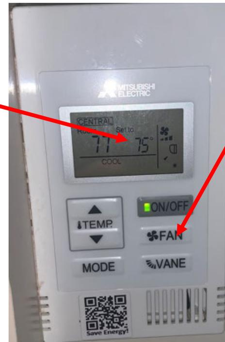
You can adjust the fan speed as well if desired, but the highest fan speed seems to work well for most spaces.
