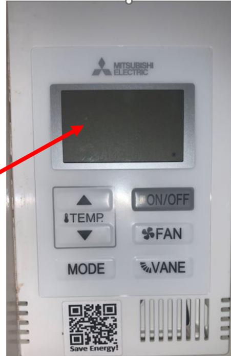
To enable cooling, press the on/off button once. The green LED will light on the button. The fan will start and the fan indicator will show on the screen. The current room temperature will show up on the screen.
