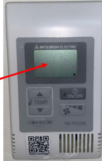
To enable cooling, press the on/off button once. The green LED will light on the button. The fan will start and the fan indicator will show on the screen.
